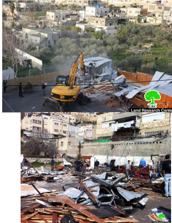
Demolition of park cultural café in Wadi Hilweh (February, 2012)
